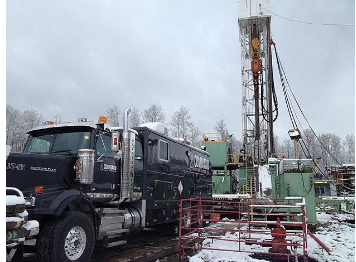
Wireline assembly hoisted by crane or derrick
